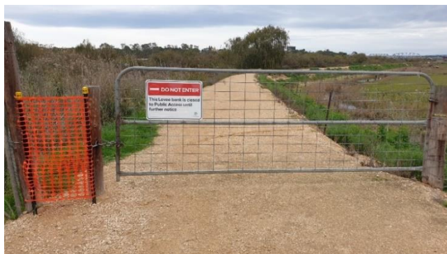
Photo: Restricted access to levee banks.
